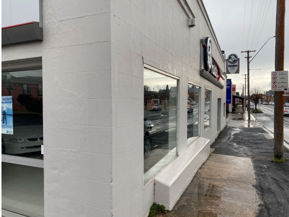
Figure 2 Western elevation of subject site (Rouse Street).
