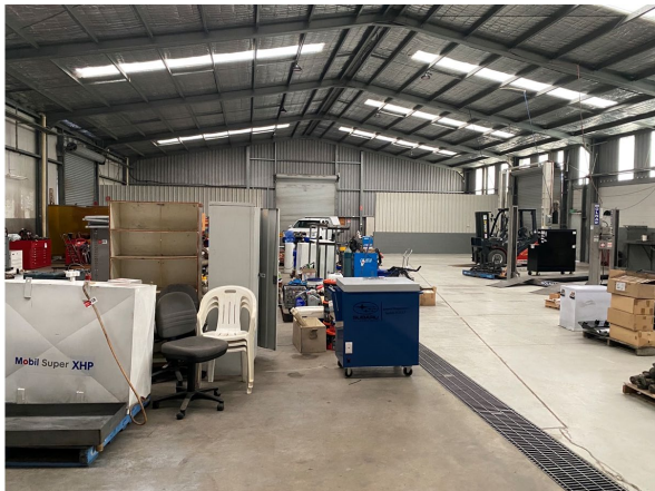
Figure 14 Interior fabric of rear warehouse.
