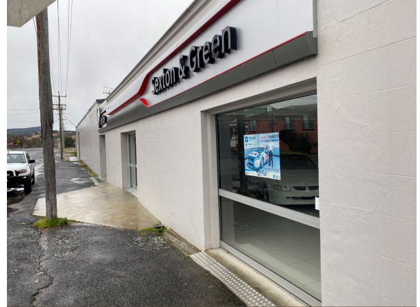
Figure 3 Western elevation of subject site (Rouse Street).
